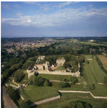
An aerial view of Carisbrooke Castle, showing its proximity to the coast.
