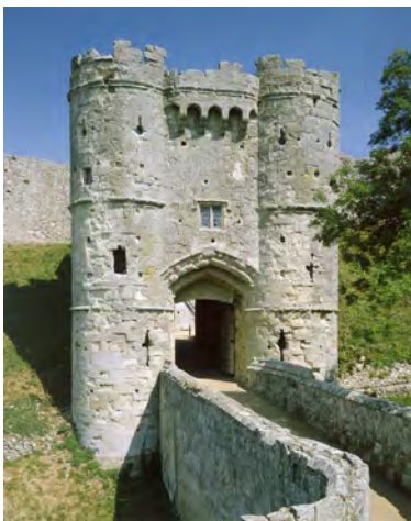
The gatehouse at Carisbrooke Castle.
