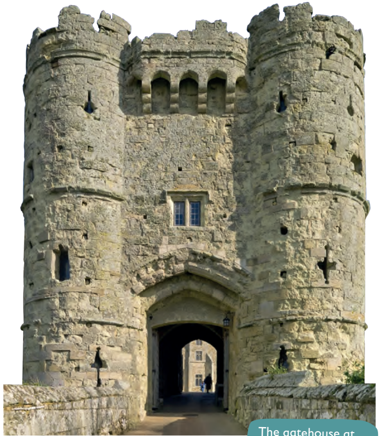
The gatehouse at Carisbrooke Castle.
