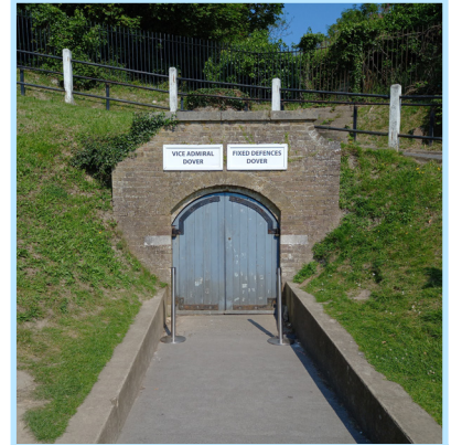
Secret Wartime Tunnels entrance.
