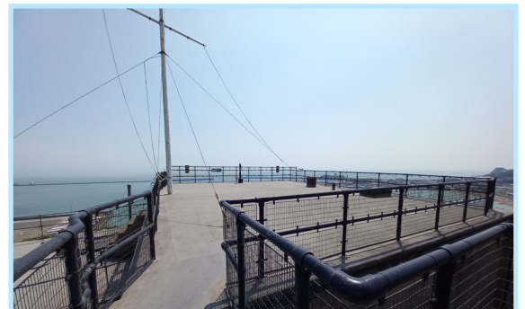
The roof of the Port War Signal Station.
